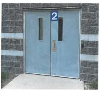
**F-409.5.6 Exterior access to rooms:** Doors that provide access directly into a room shall be marked with the room number or descriptive name per section 409.4.1 directly below the exterior door identification number.
