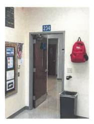
F-409.4.3.2 Ingress/Corridor side of door. Room numbers shall be placed above the door and shall be readable from all angles from the hallway or area to which they open. The numbers shall be in white on a background of the zone color. Each character shall be not less than 4 inches (102 mm) high with a minimum stroke width of 1/2 inch (13 mm).
